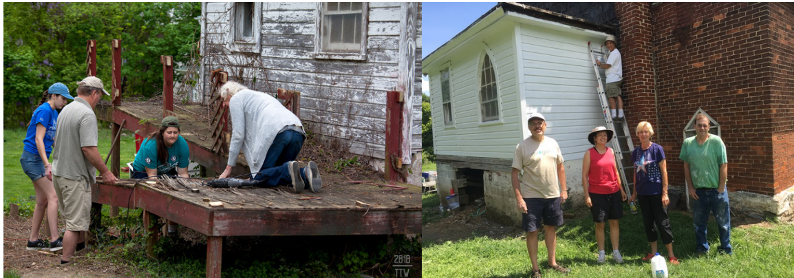
On the cover: Preserve WV AmeriCorps members conduct a civic service project on behalf of the Harpers Ferry-Bolivar Historic Town Foundation. Lauren Kelly, the AmeriCorps member serving with the Jefferson County Historic Landmarks Commission, organized volunteers and helped to plan and execute this project, which involved removing a non-ADA-compliant handicapped ramp and painting at the vacant, former First Zion Baptist Church. Built by volunteers in 1893 as a church and school, First Zion was a gathering place for African-Americans in Harpers Ferry and nearby Bolivar. It is now owned by the Harpers Ferry-Bolivar Historic Town Foundation, which plans to turn it into a community center that includes interpretation of the area’s African-American history. This evaluation studies the impact of AmeriCorps member service on visitors to museums and historical sites, but it does not capture this other, essential role Preserve WV AmeriCorps members serve: helping saving many historical properties themselves.
