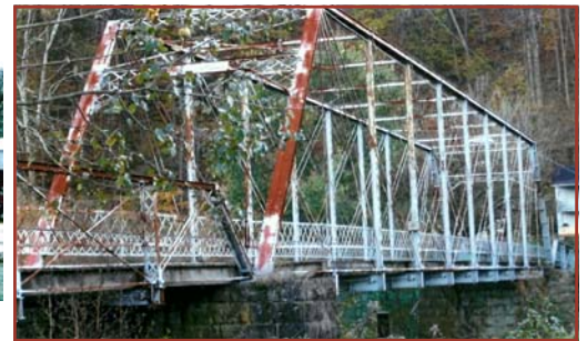
Old Glenville Bridge – GLENVILLE
