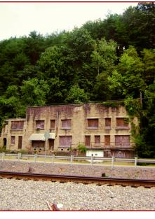
Alec Deminio, this building stands two stories tall and originally served as the town's general store. After standing vacant and abandoned for decades, the flat roof has collapsed and the entire building is in very poor condition. However, the Coalfield Development Corporation has plans to acquire, revitalize, and adapt it for use as the headquarters for its *21st Century Jobs Initiative*, a
