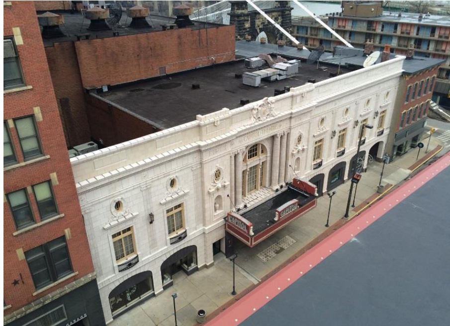
In late 2014, the restoration of the Capitol Theater façade was completed.
